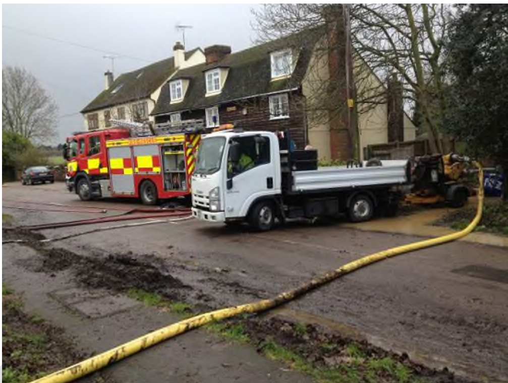
Figure 2: Emergency pumping of flood water
