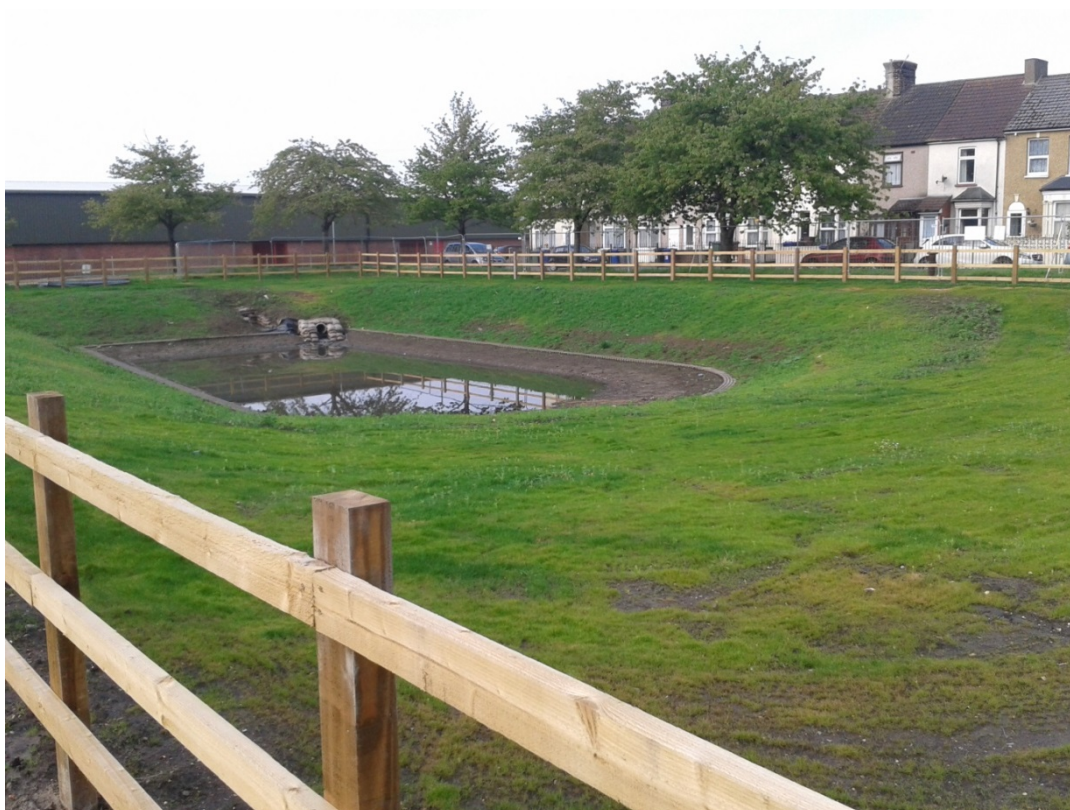
Figure 1: Drainage Pond at Gumley Road
